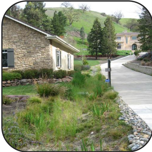
Large Residential Rain Garden
